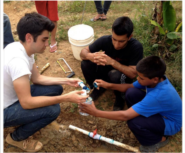
Applying PVC primer to pipe with youth in the community. August 2014; Pinalito, DR.
